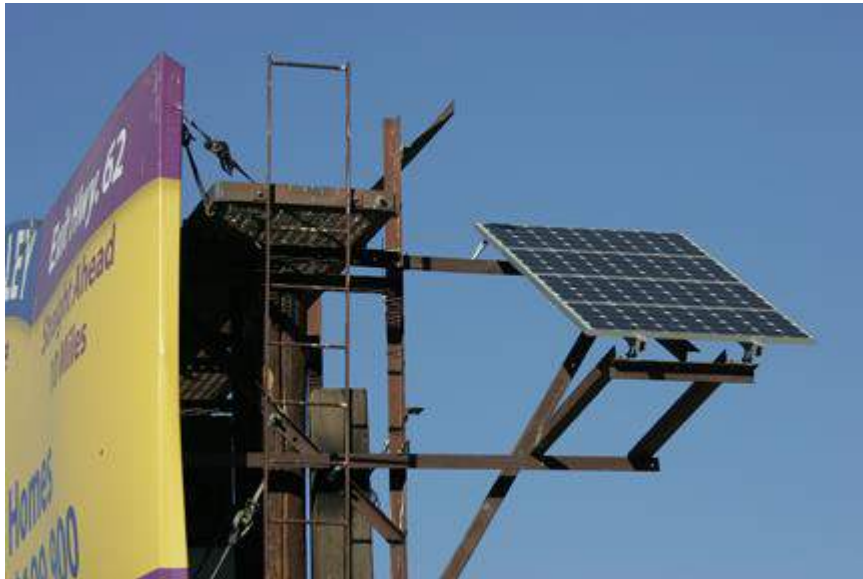
Figure-1: Solar powered light for Hoarding
