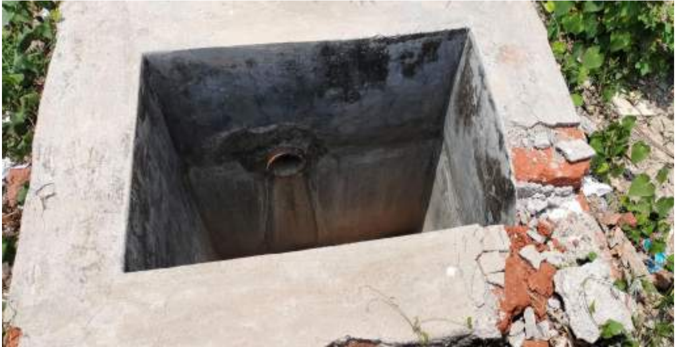
Photo-6: View rain water collection from building
